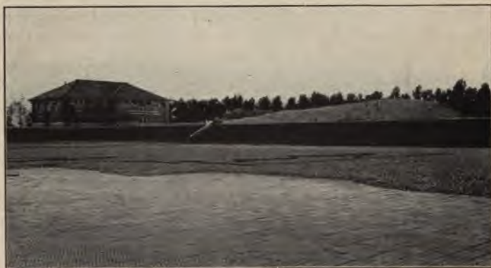
FILTER BED OF THE INDIANAPOLIS WATER WORKS.
